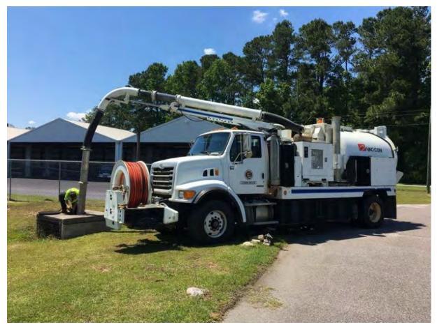
Figure 3-7: Catch Basin Maintenance Operation
