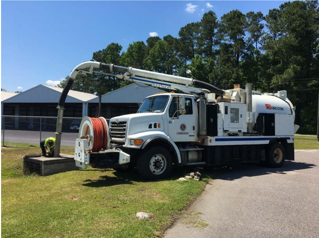
Figure 3-7: Catch Basin Maintenance Operation
