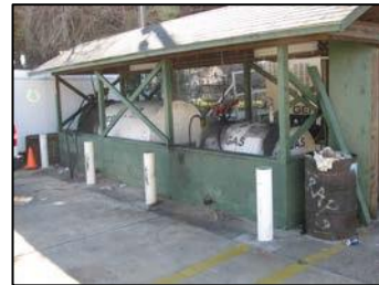
Covered/Contained Fuel Tanks
